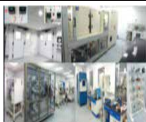
Figure 50 : Dehumidified room's external internal views.
